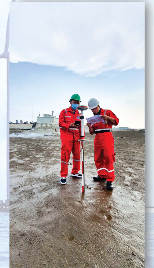
Inspection for buried cables at landing zone
